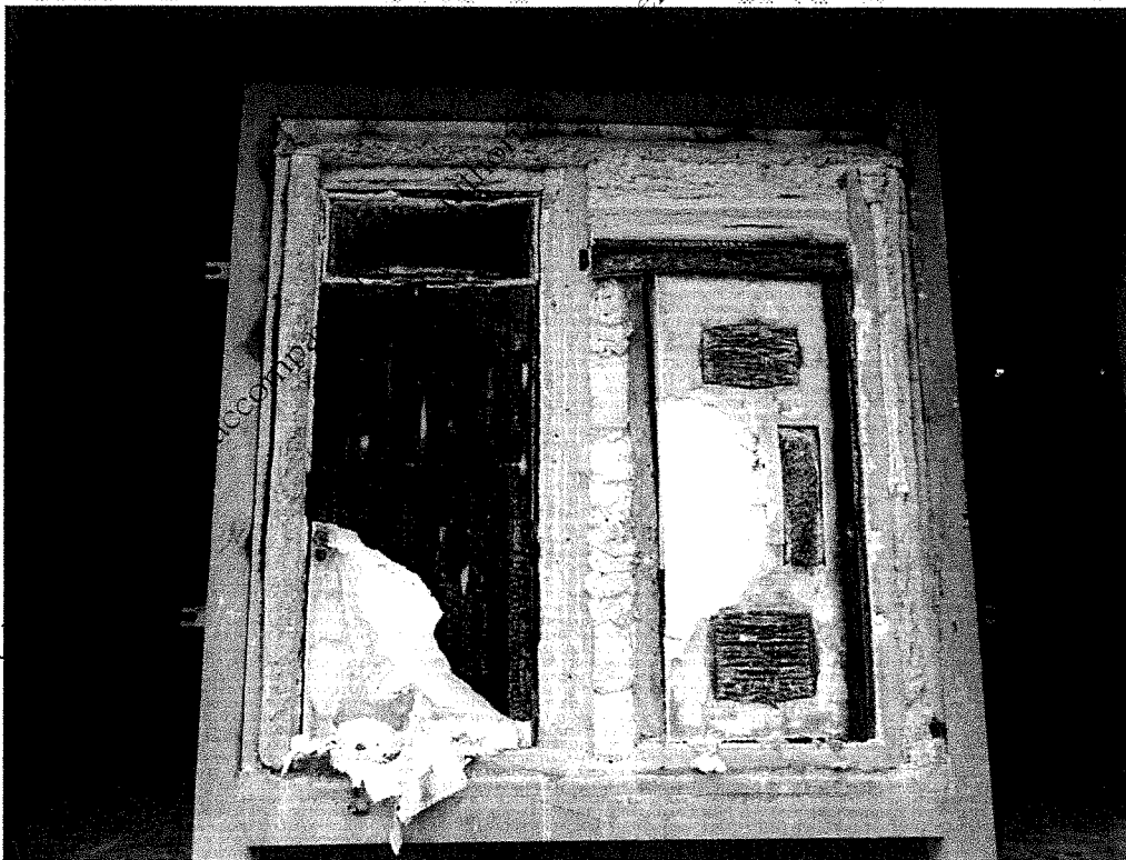
Photo 6. Exposed surface of the specimens at after test. (Left: Door B; Right: Door A).
